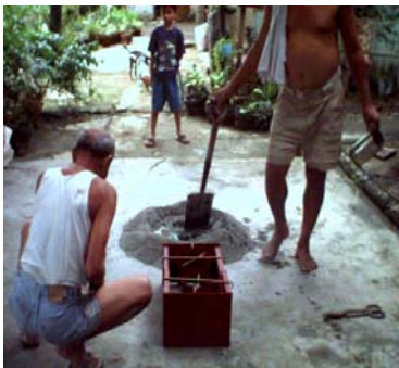
Mixing Concrete
