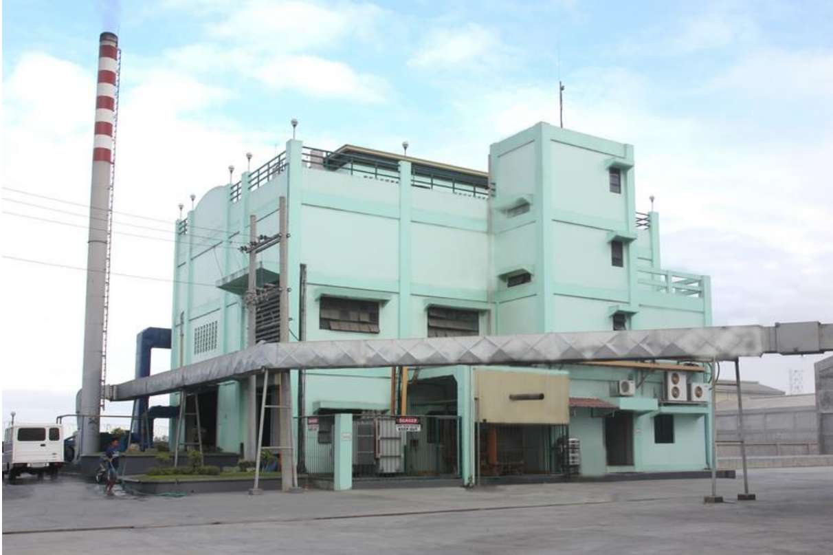
Figure 4-11: Family Choice Rice Husk Power Plant [13]
