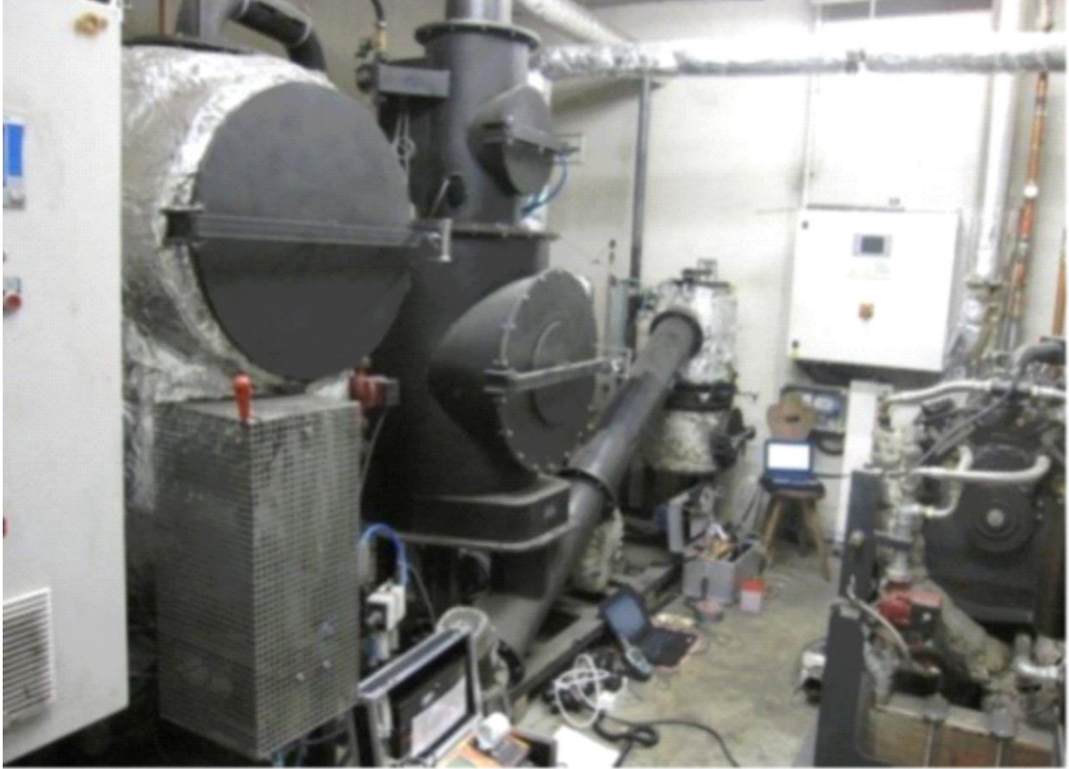
Figure 4-2: Spanner gasification system in Austria [5]
