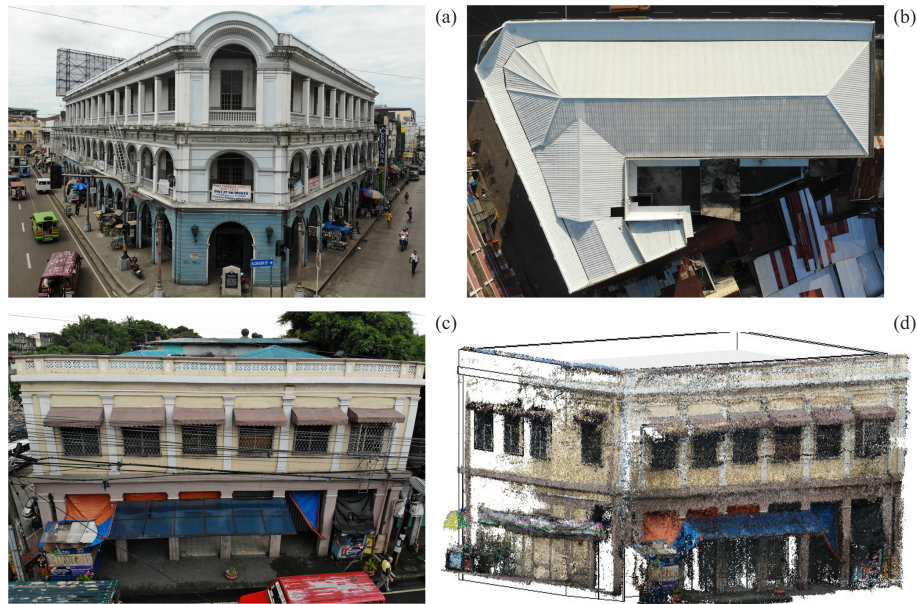
Figure 6. Use of new technologies for the survey of the Iloilo City CH assets: Villanueva building front façade (a), and roof (b) by drone; Villanueva building 6 front façade (c) and point cloud (d) by drone and photogrammetry respectively.
