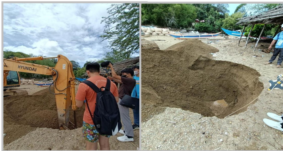
Open Test Pit Method
